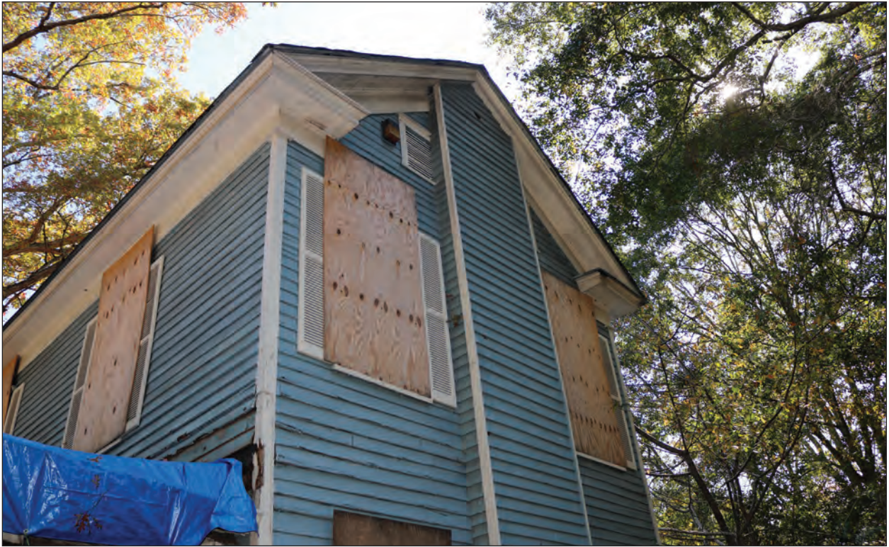
A. Detail of Corner Pilaster and Cornice Returns, Facing Southeast
