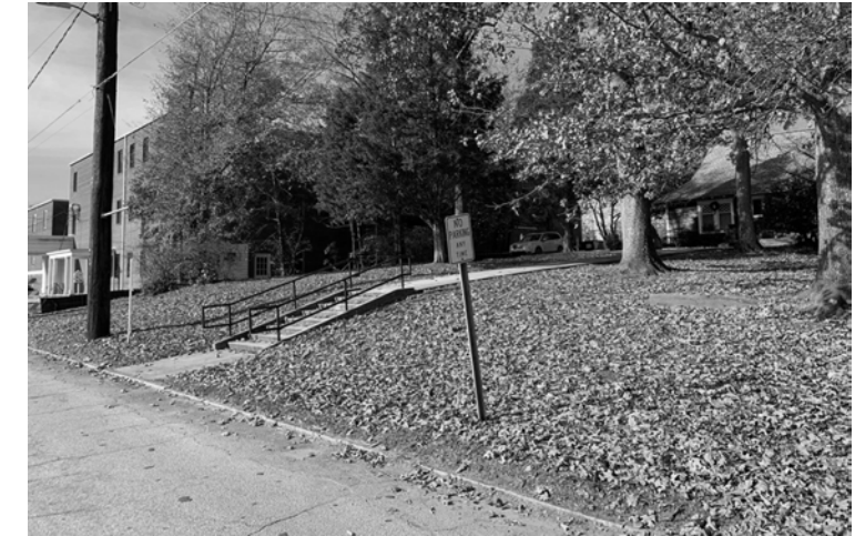
EXISTING STAIRS AT WOMENS BUILDING
