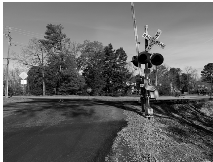
2. EXISTING FROM CHURCH STREET AT RAILROAD CROSSING
