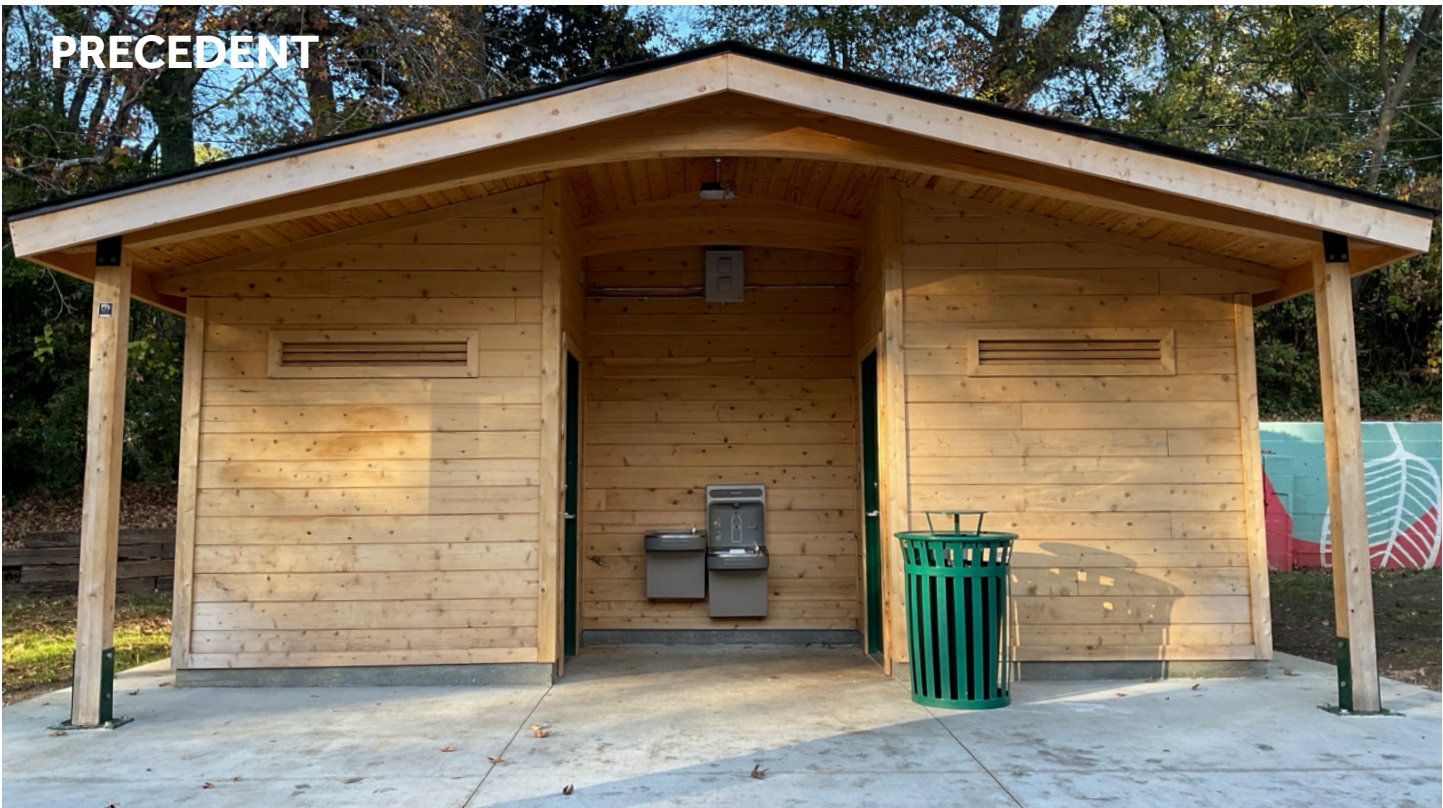
BELOW New prefabricated bathrooms installed in the City of Doraville in 2024 helped save installation costs across multiple parks.
