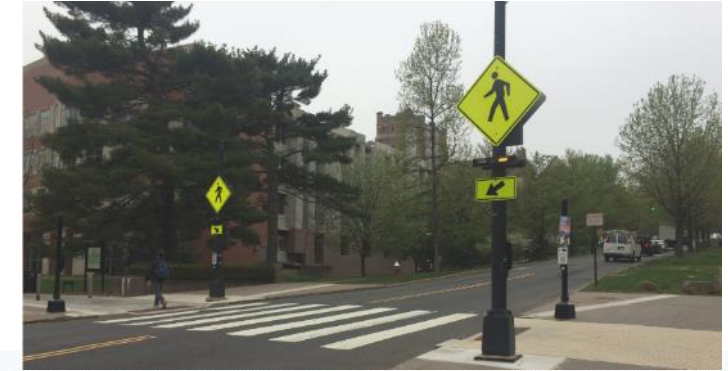
Rectangular Rapid-Flashing Beacon
