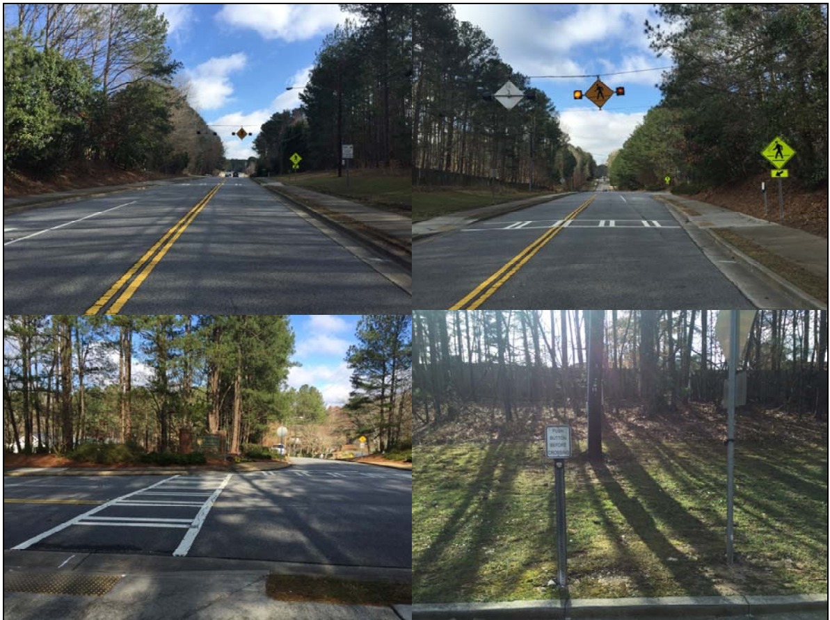
Figure 6 - Example of Pedestrian Crossing with Wig Wag Flashers Active by Push Button
