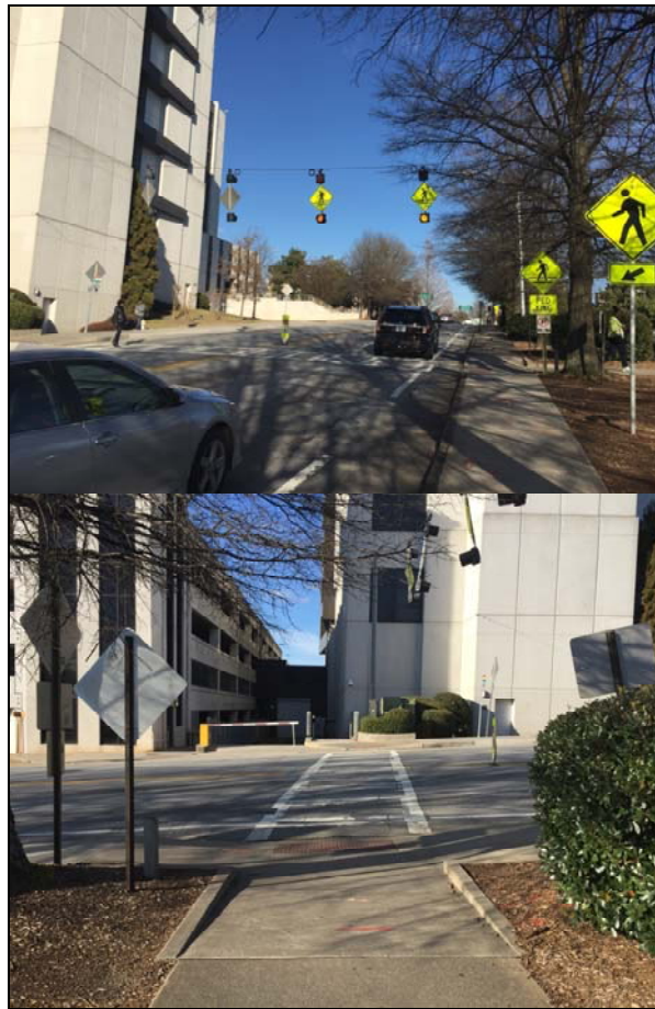
Figure 5 - Example of Pedestrian Crossing with Continuous Wig Wag Flashers
