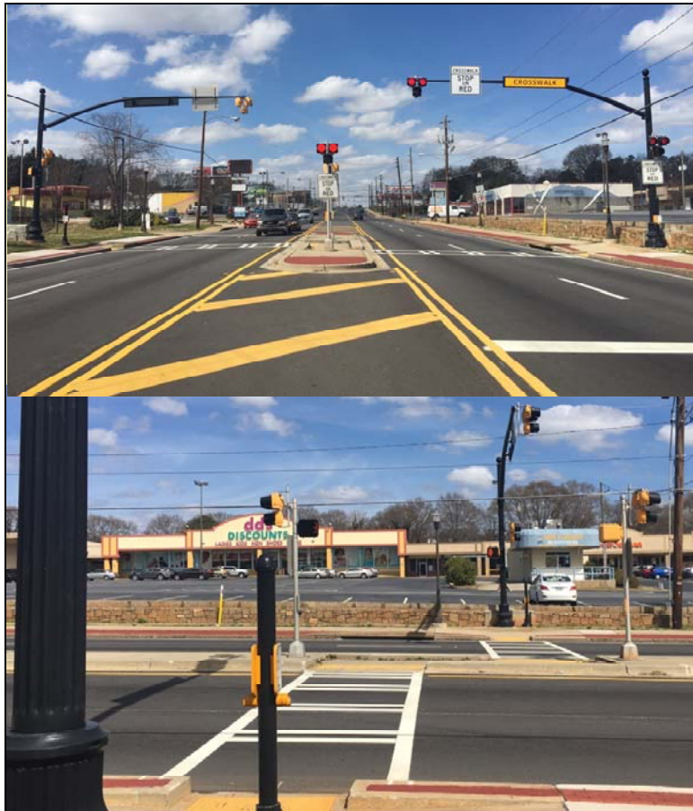
Figure 8 - Example of Pedestrian Crossing with Hawk Signal
